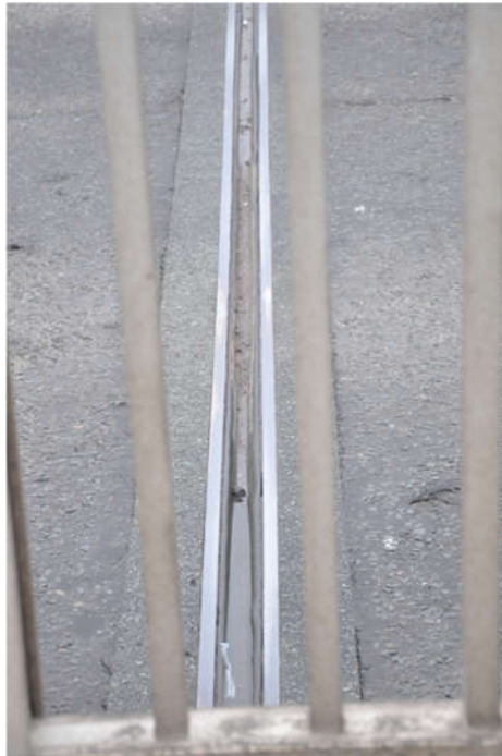
Figure 4-3 Typical expansion joint on Tay Road Bridge
