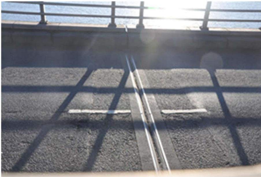
Figure 7-17 Normal expansion joint style of No. 1-29 and 34-42
