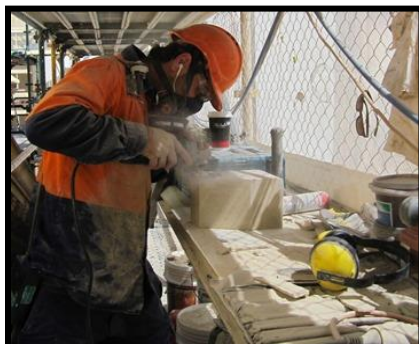
Figure 2: 'Spinning' with angle grinder
