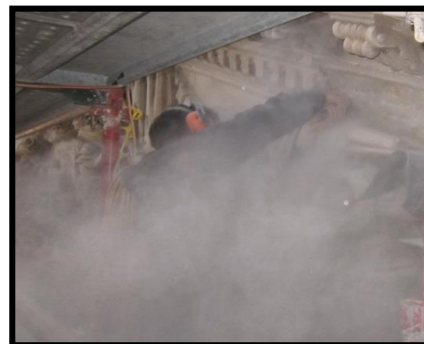
Figure 3: 'Chopping out' with grinder
