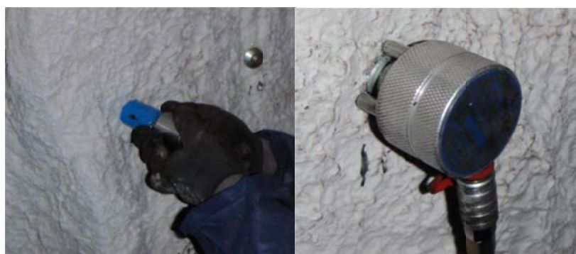
Figure 3: In situ adhesion strength test (a) overcoring, (b) dolly under test
