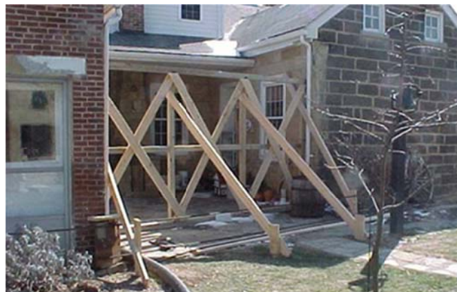
Figure 4: Mitigation Measures for a Historic House Located over the Central Portion of a Longwall Panel
