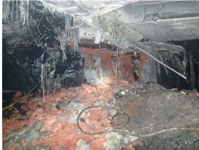
Figure 13: Recovery of shield 76 from within the consolidated muck pile
