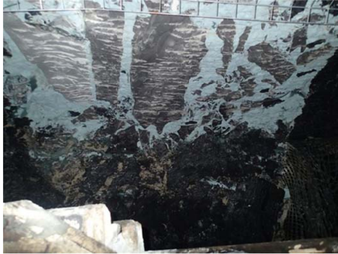
Figure 12: Consolidated muck pile and grout filled voids
