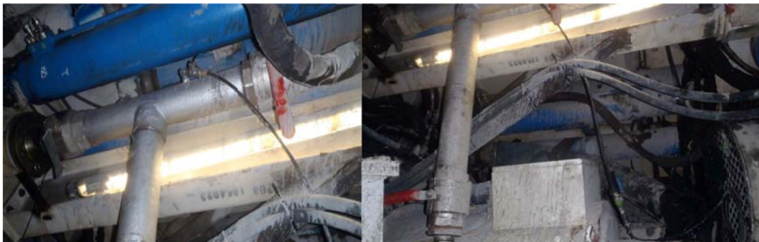
Figure 11: Methane sampling/bleed hose (left) behind the cutter bulkhead (right)
