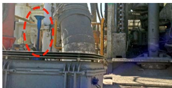
Figure 3: Dust monitor in use during drilling operations
