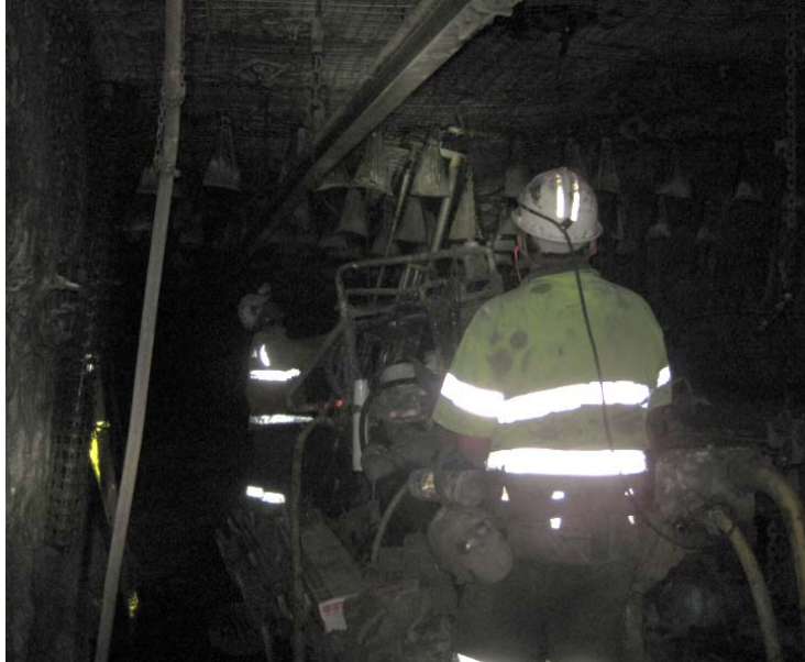
Figure 8: Current cable bolt drilling practice is manual-handling intensive
