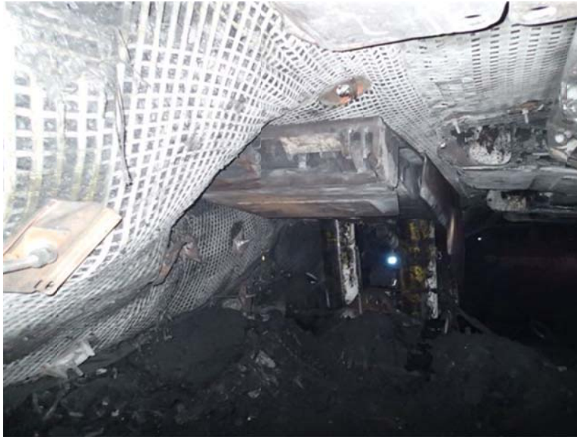
Figure 5: Shield 76 under the fall – in the middle of the face road
