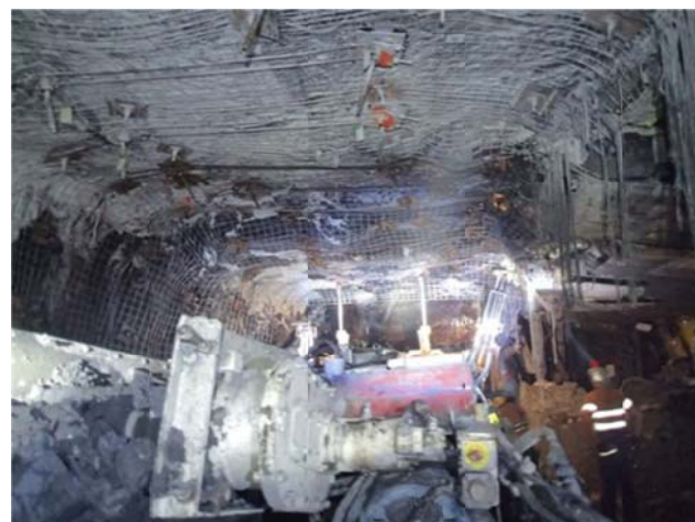
Figure 11: Roadheader re-mining through the consolidated muck pile under the backfilled void
