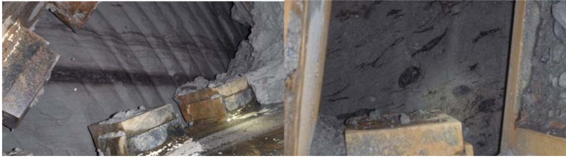
Figure 10: Typical coal lenses (Left) and cutting face (right) of a TBM with specs of coal.
