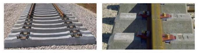
Mono Block Concrete Sleepers
