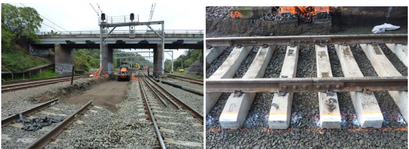
Figure 9: Installation of USPs at GIJs
