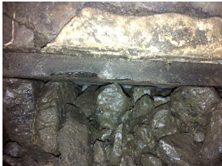
Figure 13: USP and ballast inspection
