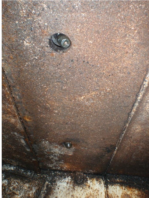
Figure 7.15 Mine A Installed Sprays Before Crusher
