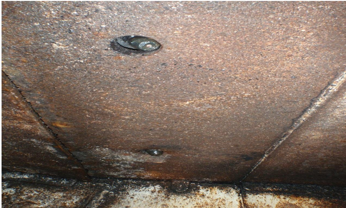
Figure 4.5 Typical Hollow Cone Sprays inside the Crusher
