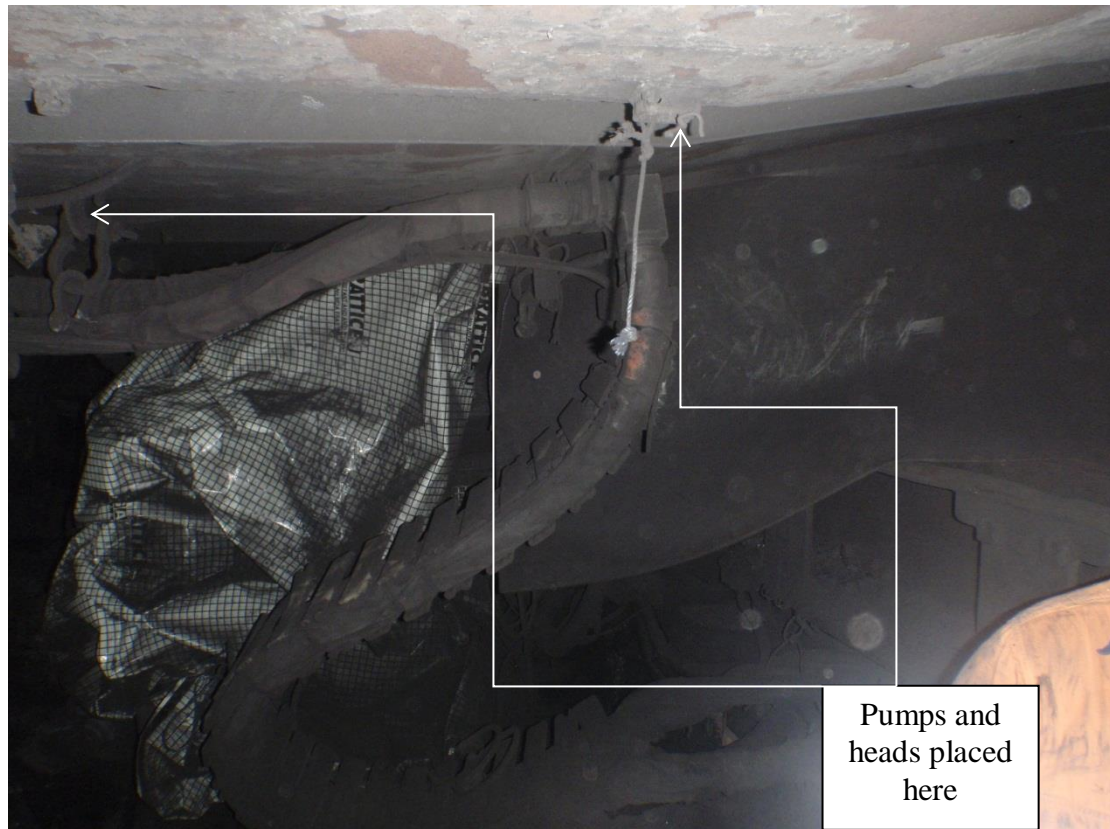
Figure 7.9 Mine A Pump and Head Location in the Tailgate
