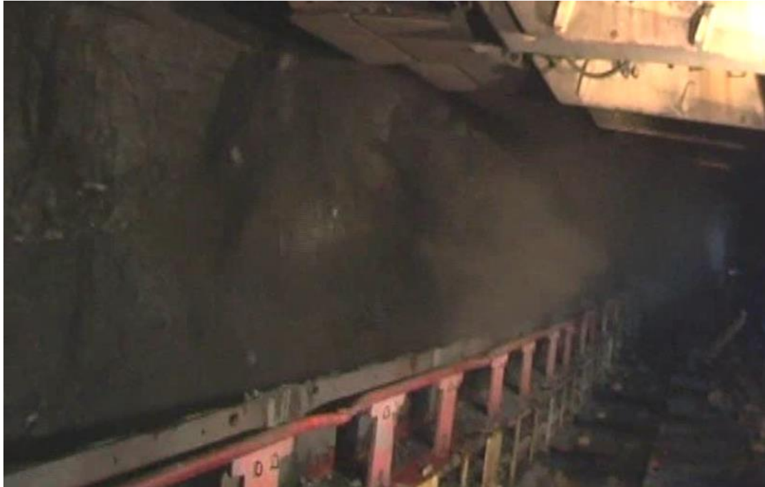
Figure 3.7 Dust Being Entrained into the Walkway from Raised Drum
