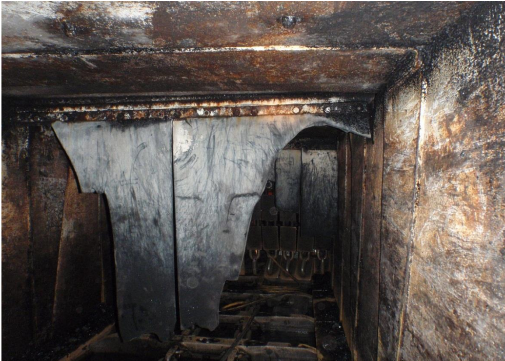
Figure 4.2 Conveyor Belt Strips inside the Crusher before the Hammers
