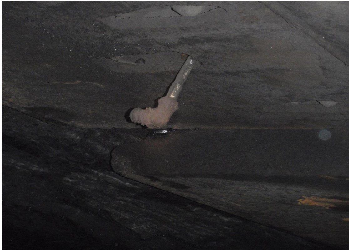
Figure 7.21 Mine A Installed Chock Sprays
