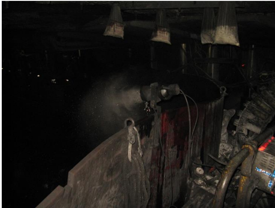
Figure 4.16 Venturi Spray Installed on BSL Maingate
