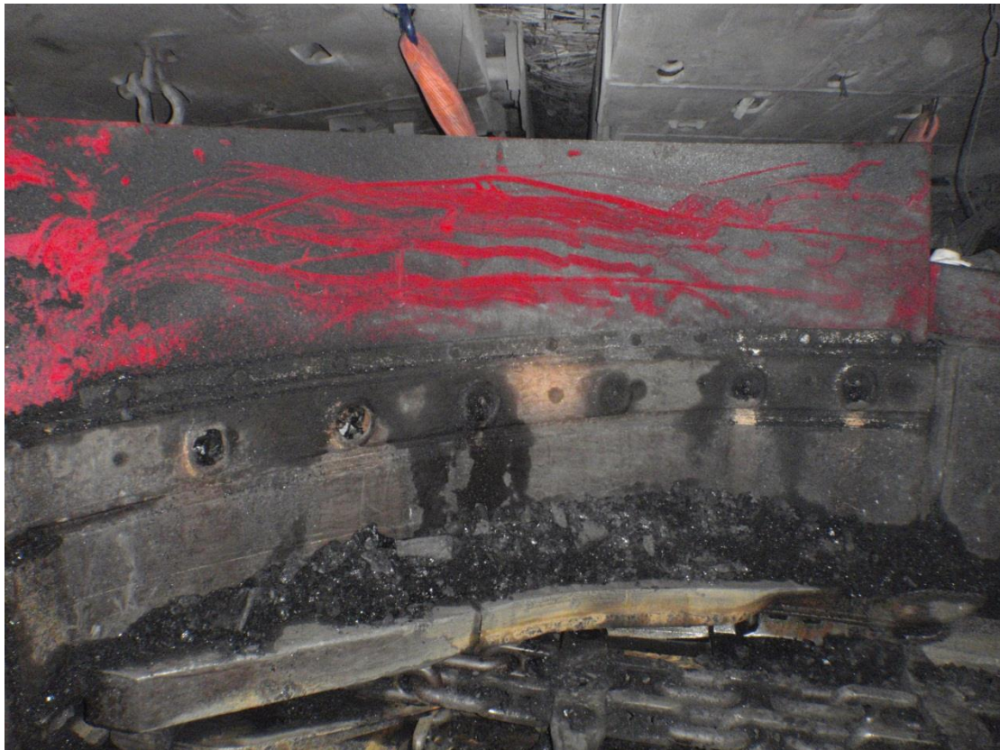
Figure 4.4 Typical Spray Setup to Suppress Dust from the Face to Crusher Intake
