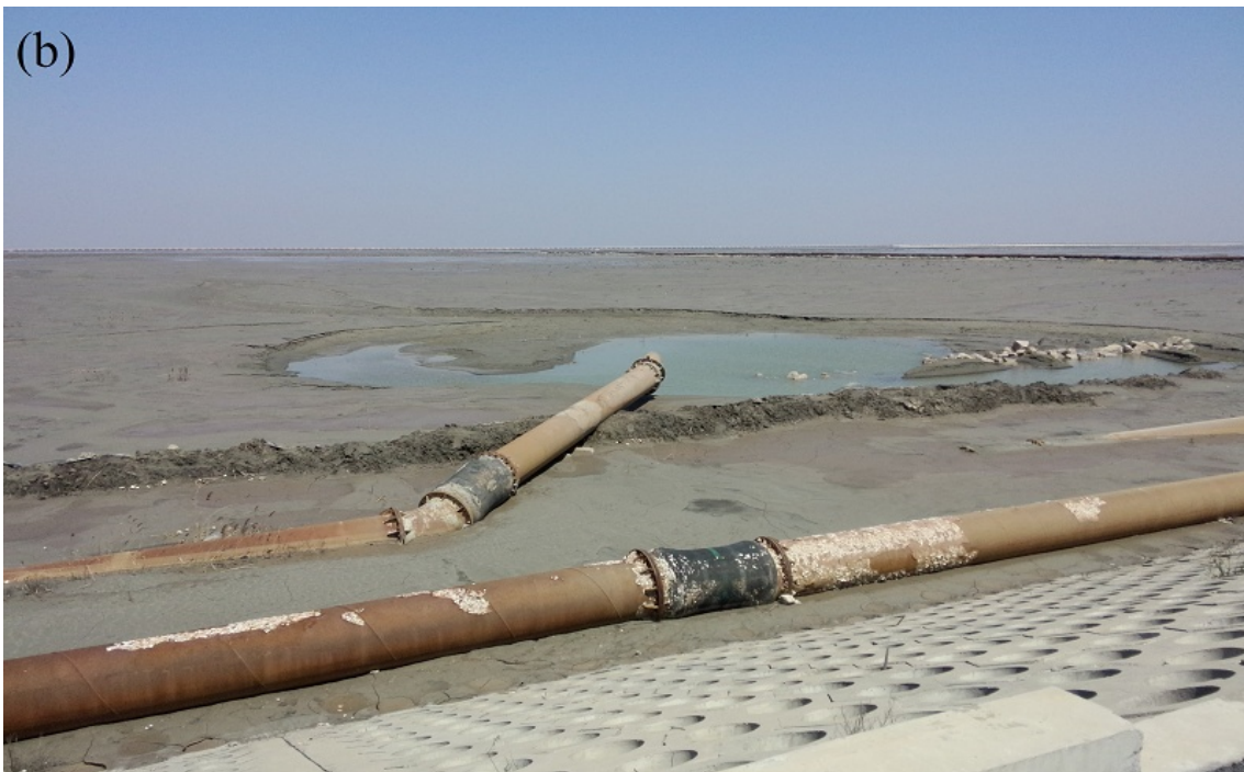
Figure 2 Project site reclaimed filled with non-solidified dredged soils (a) Part of reclaimed land for Hengsha east shoal reclamation project; (b) Project site for current study
