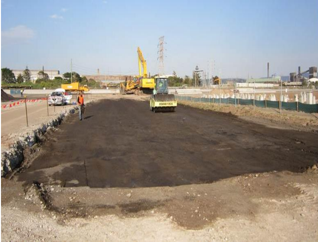
Fig. 23 Port Kembla construction site: during compaction [45].
