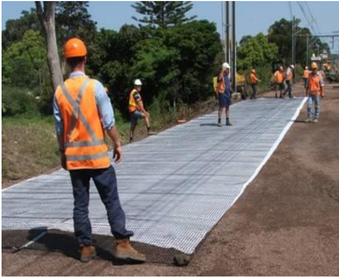
Fig. 10 Installation of geocomposite at Bulli.
