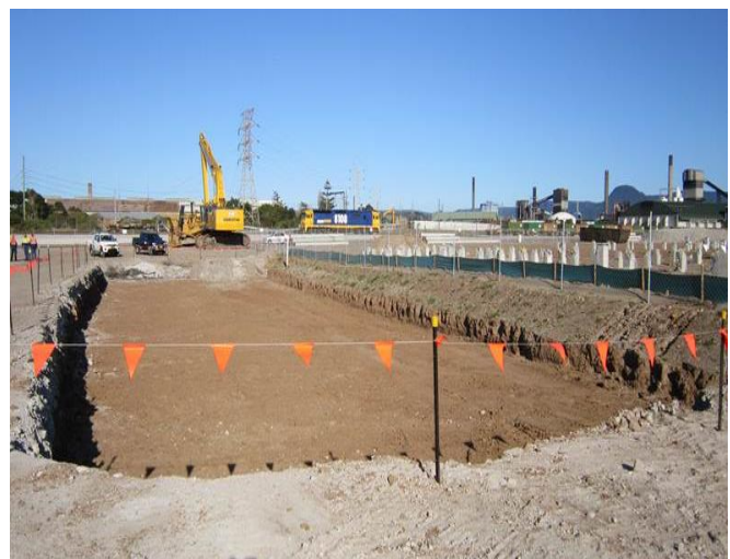
Fig. 22 Port Kembla construction site: prior fill placement [45].
