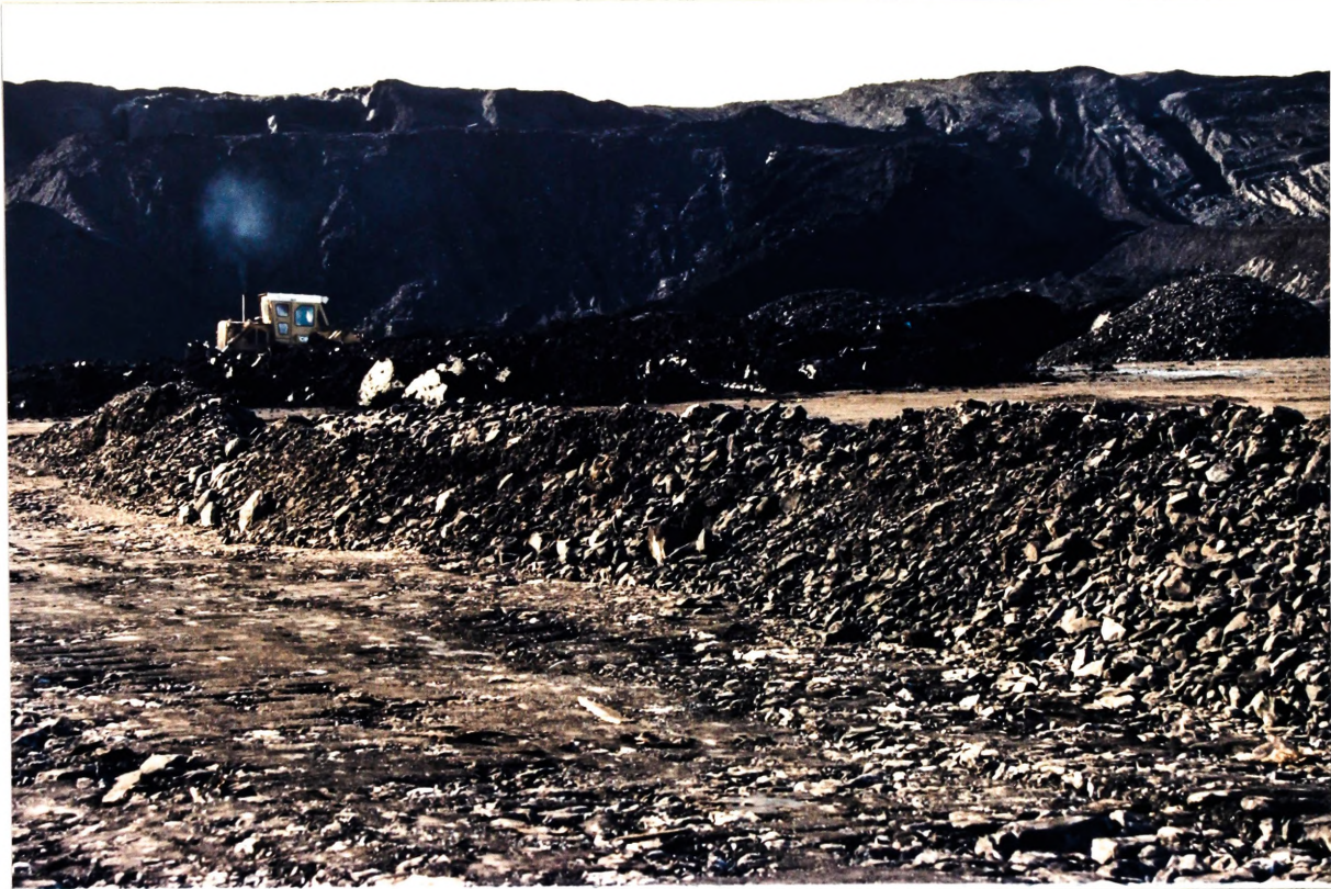
Figure 2.7: Uphill Technique of Stockpile Construction Using Horizontal Layers
