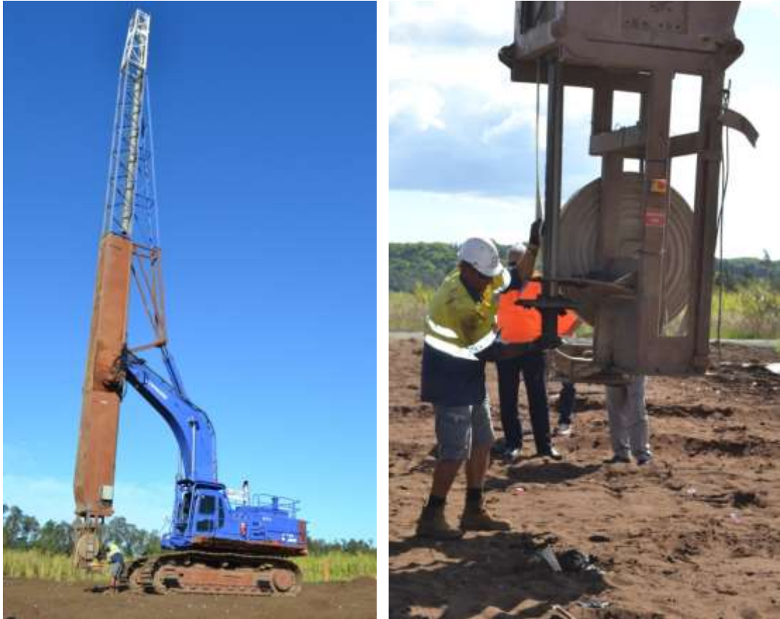
Figure 2.7 : Drain Installation equipment.
