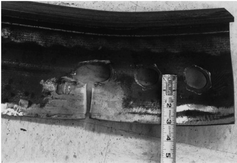
Figure 4 Tee section bolted at the web failing in block shear [10]
