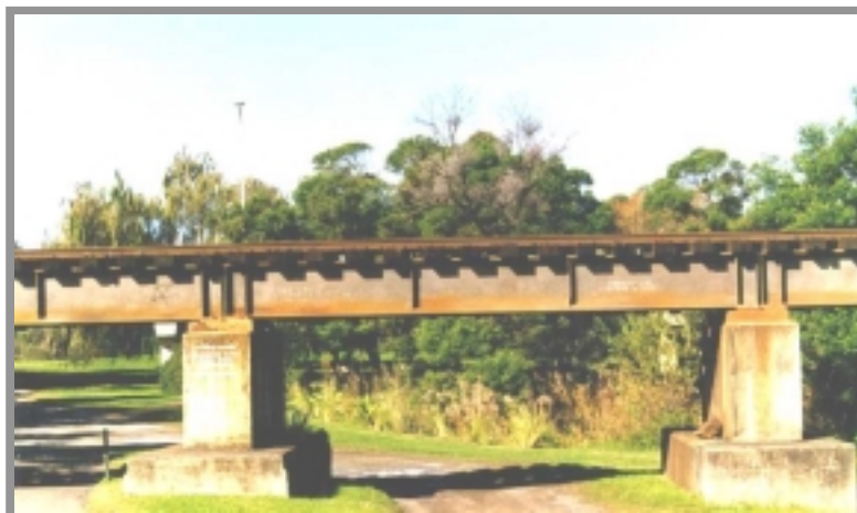
Figure 3.1.2. Typical Mullet Creek Railway Bridge approach span.
