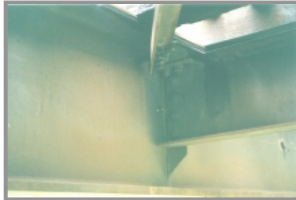
Figure 3.1.6. Cross girder and sway bracing connections.
