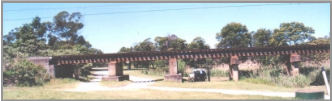
Figure 3.1.1. Mullet Creek Railway Bridge.
