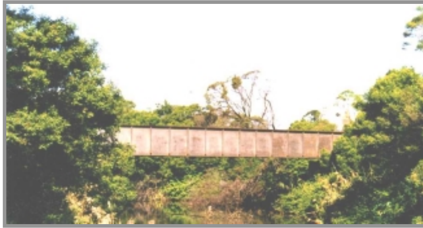
Figure 3.1.3. Mullet Creek Railway Bridge main span.
