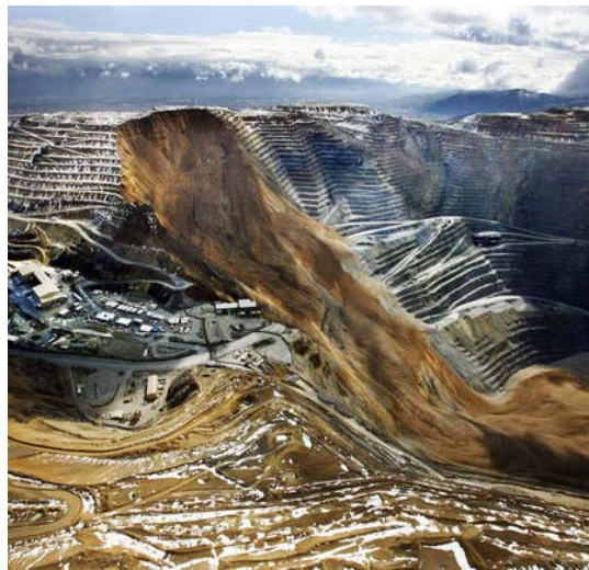
Figure 1: Slope instability causing landslide, Bingham Canyon (Pankow et al. , 2013)
