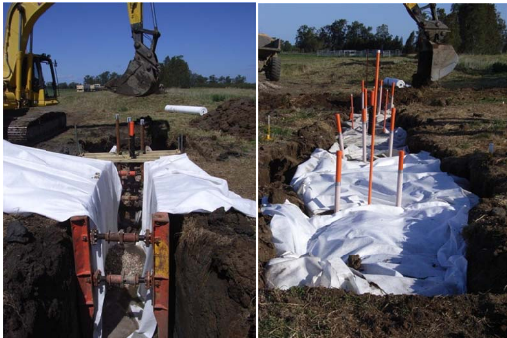
Figure 4.3 Installation of PRB at the study site
