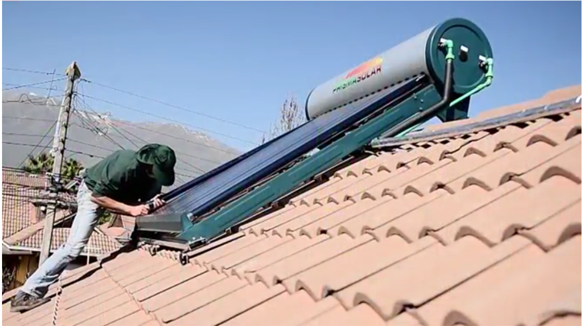
Figure 79: Installation of a Solar Thermal Collector
