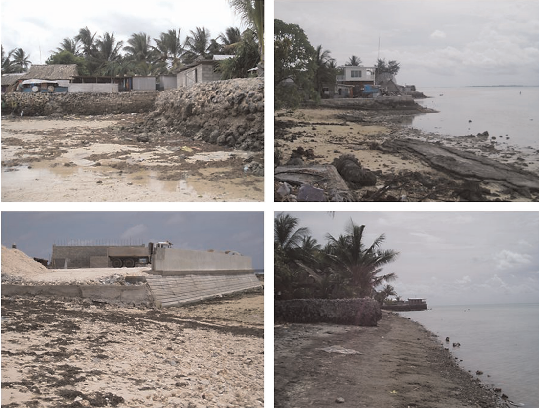
Atolls, Figure 9 Human impacts on atoll shorelines, illustrated with examples from Tarawa Atoll, Republic of Kiribati: top left , Oceanside seawall at Nanikai, which reduces access to the ocean; top right , private reclamation; lower left , large reclamation for Mormon Church, Bairiki; lower right , private reclamation that has resulted in erosion of shoreline.
