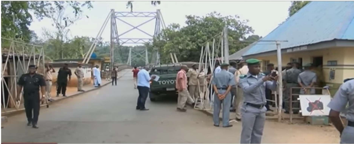
Picture 6 - Mfum Border Bridge (Nigeria Side) 18
