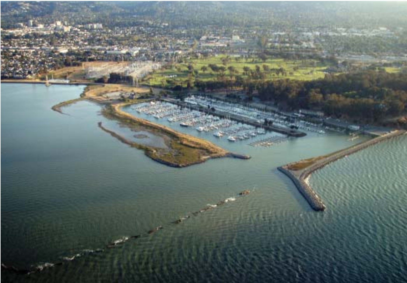
A Marina and Golf Course sit along the San Francisco Bay. The Coyote Point Marina, the Poplar Creek Golf Course and a power substation are just some of the uses for the heavily developed shore along the San Francisco Bay near San Mateo, California. © Gerick Bergsma
