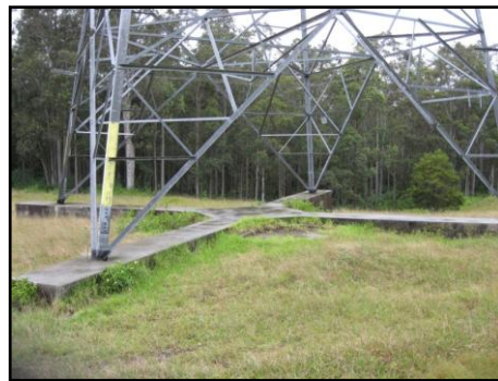
Figure 16 - Cruciform footings installed under the TransGrid 330 kV suspension towers in the early 1980's
