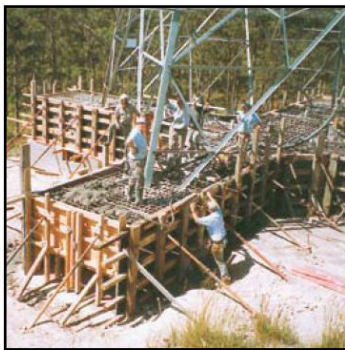
Figure 16 - Cruciform footings installed under the TransGrid 330 kV suspension towers in the early 1980's
