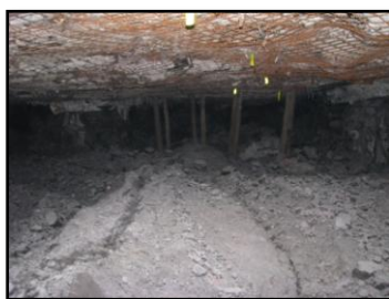
Figure 9 - Moderate floor heave in 3-North panel (outbye)
