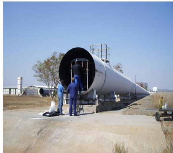
(b) At the mouth of the tunnel
