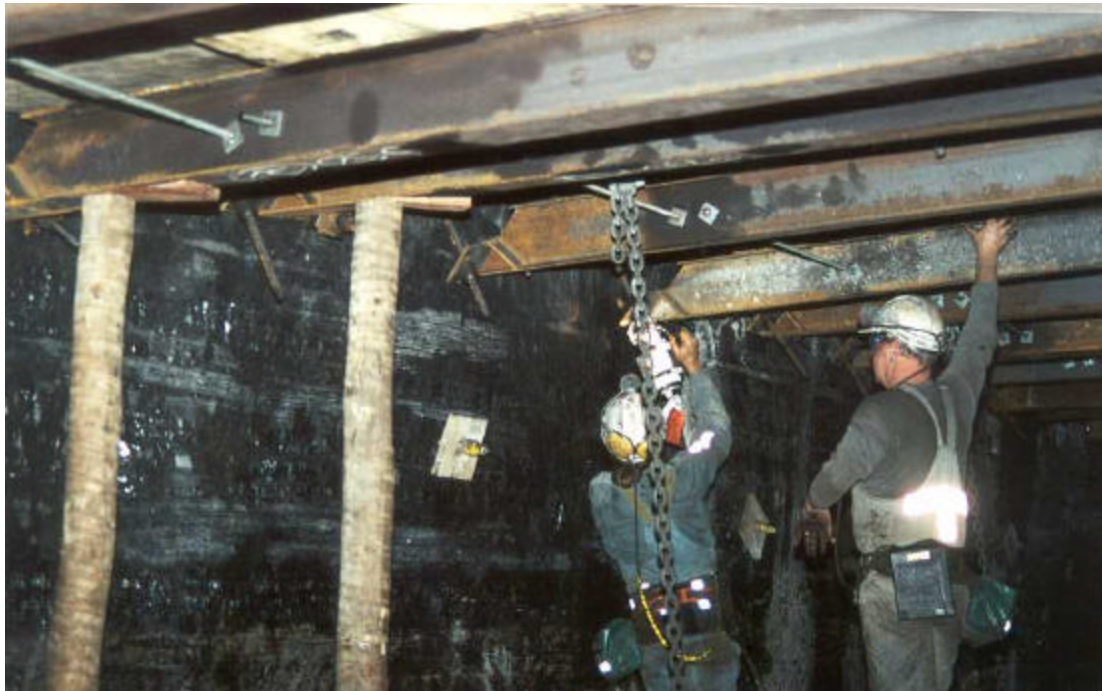
Fig 16 – Installing steel sets in the maingate LW103
