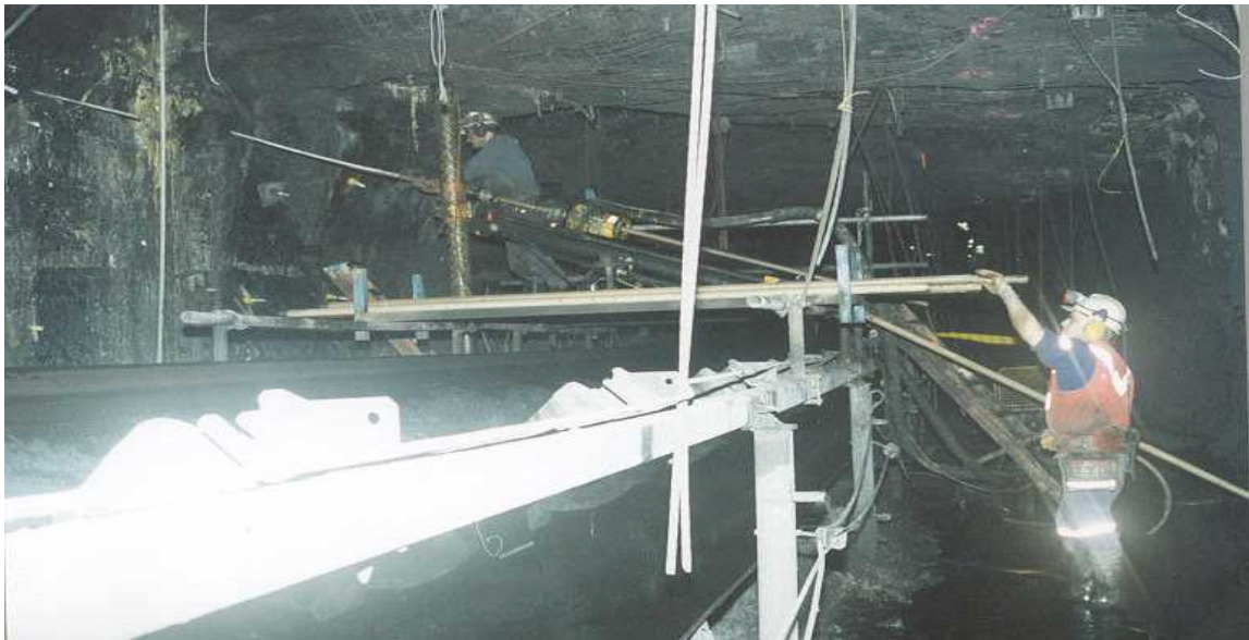
Fig 14– Drilling of the spile holes over the longwall belt. LW103
