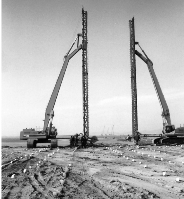
Figure 2. Typical installation rig (Source: Colbond bv, The Netherlands, http://www.colbond-gepsynthetic.com ).
