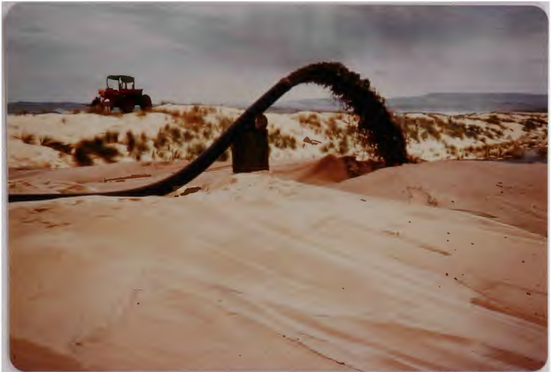
PLATE 17: Dune rebuilding by pumping dredged sand onto the dunes.
