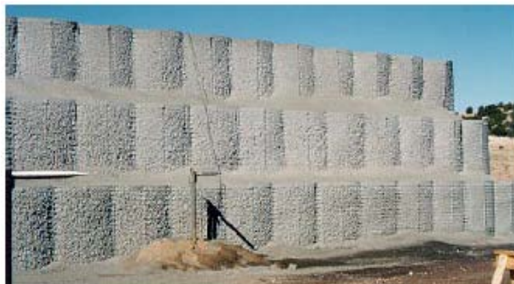
Figure 2.3: A protective barrier constructed using Hesco Bastions. (Crawford and Lan, 2006)
