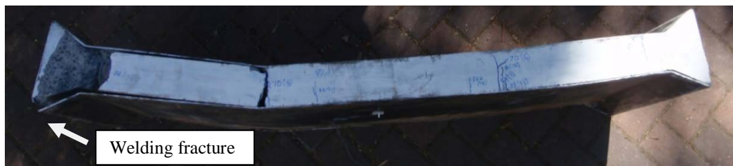
Figure 5.21: Welding fracture failure at the joint between the bottom faceplate and one of the end plates for the simply supported non-composite SCS panel under four-point bending test.
