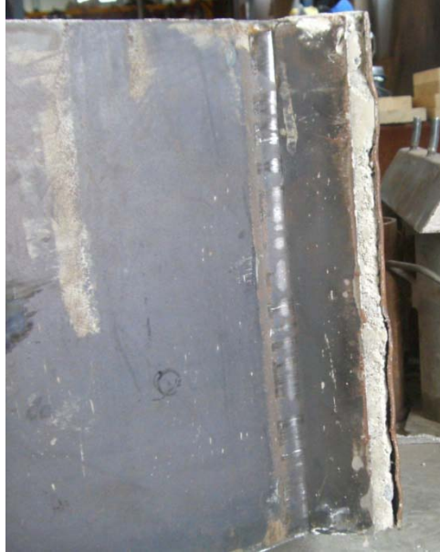
Figure 5.33: Welding fracture failure at the joint between the bottom faceplate and the end plate of the Reinforced core panel.
