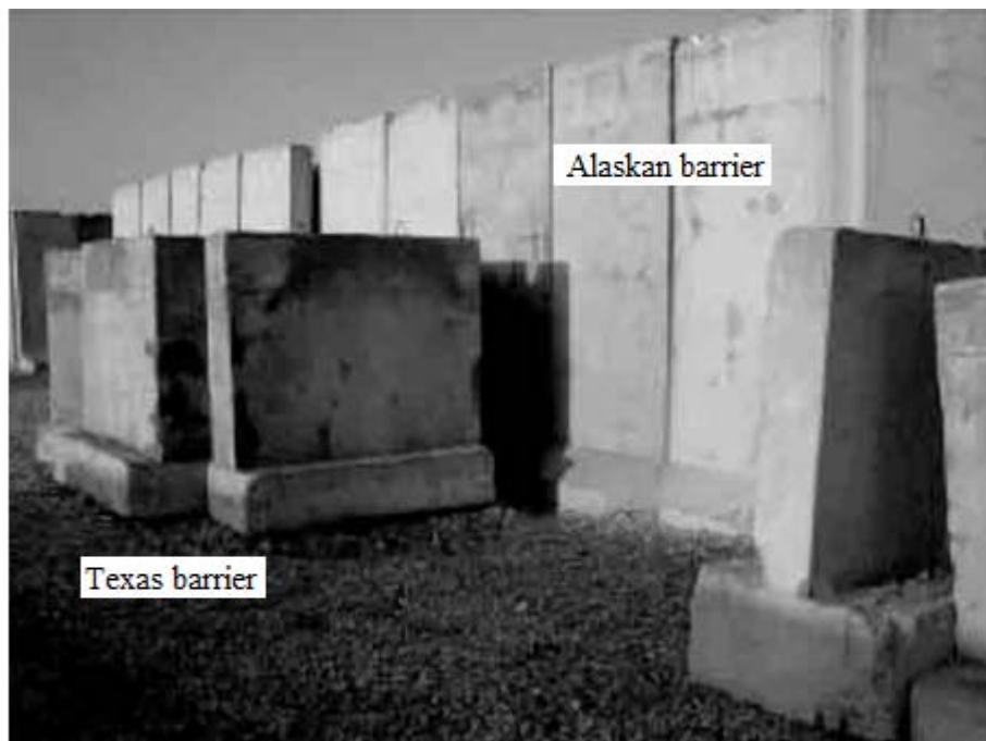
Figure 2.5: Pre-cast concrete blast walls 'Texas' (smaller in size) and 'Alaskan'. (Smith, 2010)
