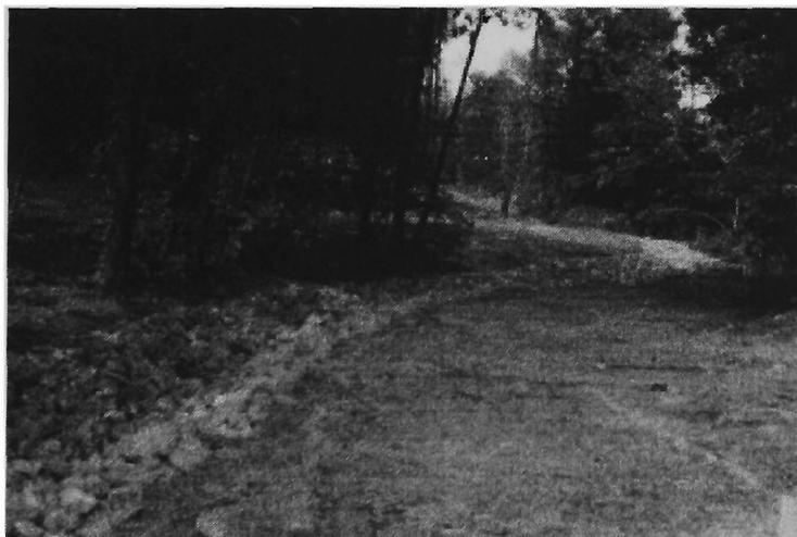
Figure 2.3. Open limestone channels for mine drainage treatment (Skousen, 2002).
