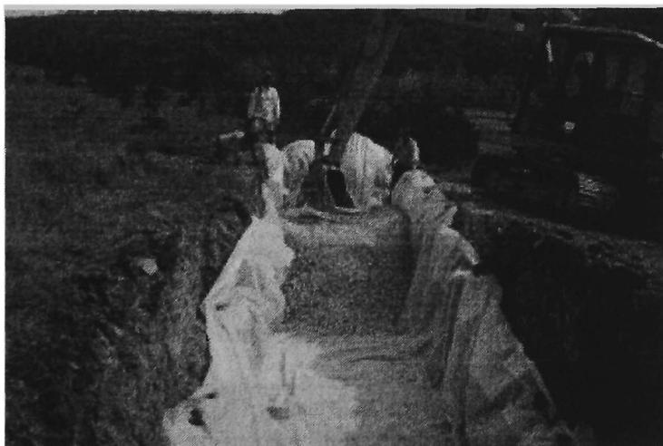
Figure 2.2. Passive anoxic limestone drains (Skousen, 2002).
