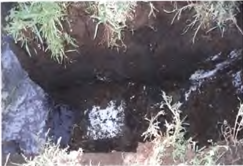
Plate 5.5: Trench showing section of lime-fly ash barrier at 1m below ground surface. Grout at upper right hand corner from an adjacent injection hole.
