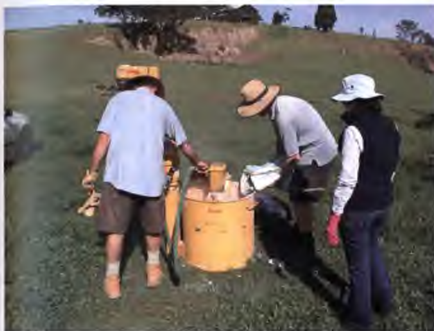
Plate 5.7: Mixing of lime-fly ash/water slurry.
