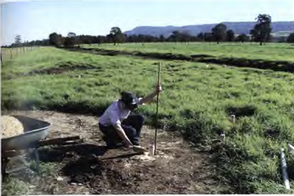
Plate 4.6: Installation of Observation Holes by the author.
