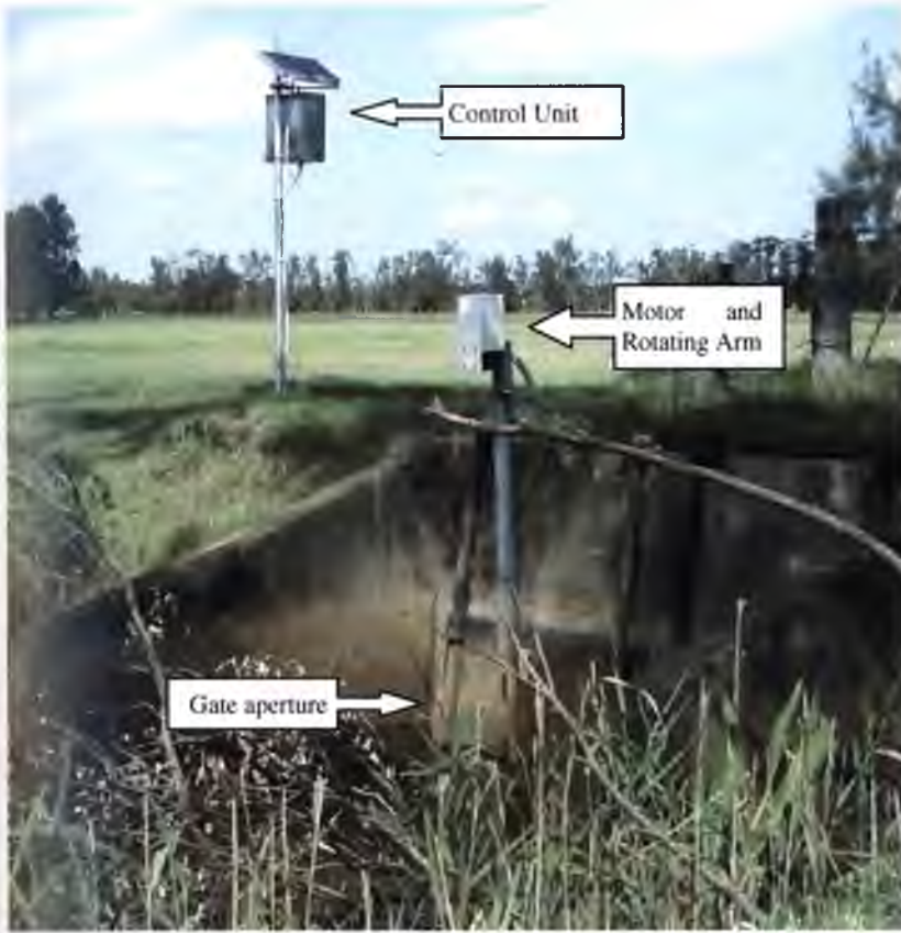
Plate 2.3: Modified two-way Floodgate
