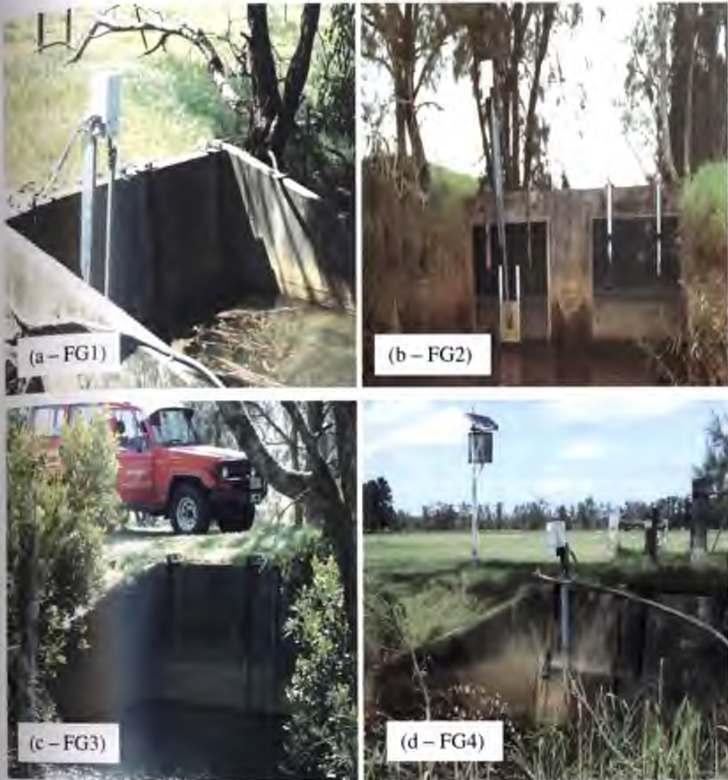
Plate 4.4: Tidal restricting floodgate installed on flood mitigation drain in the Broughton Creek Estuary. Floodgate (a - FG1), modified floodgate is located downstream from the Lime Injection Site. Floodgates (b - FG2), (c - FG3) and (d - FG4) are the other floodgates monitored during this study
