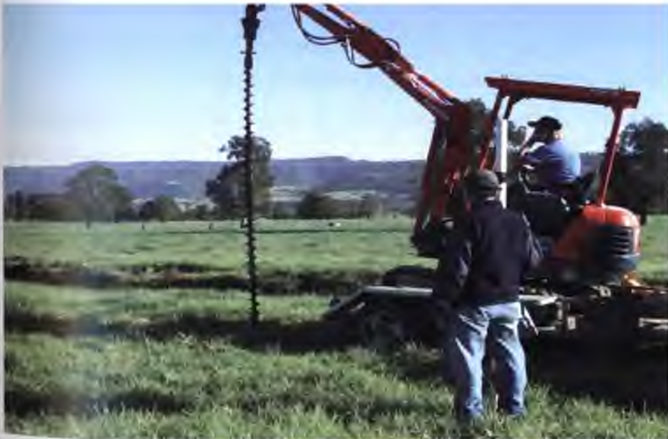
Plate 4.8: Drilling of Piezometer Holes
