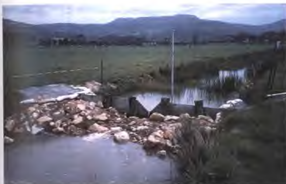
Plate 2.1: High v-notch weir
