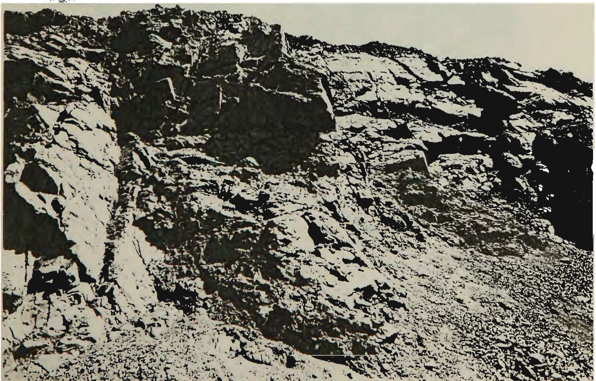
Plate 6.6 Fault-related, south-dipping jointing adjacent to the Whaleback Fault Zone.
