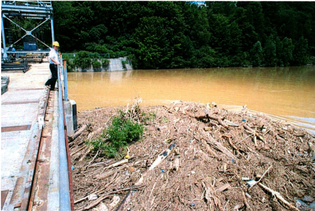
Figure 5.12: Photo of debris that was moved down Thames River and caused buildup behind Springbank Dam (UTRCA, 2000)
