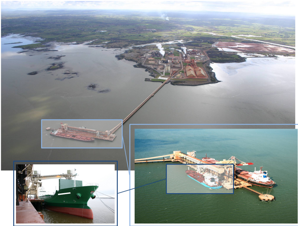
Figure 2: Aerial view and detail of the jetty and port terminal.
