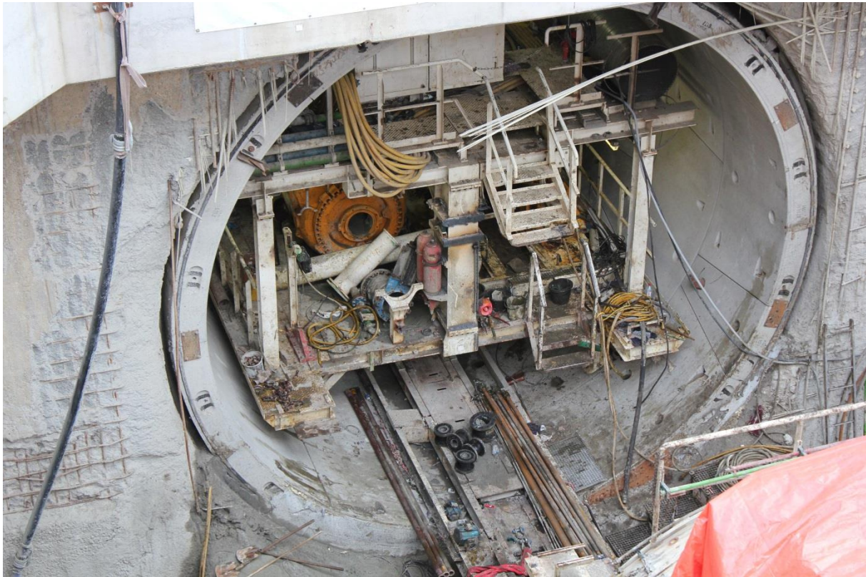
Figure 6-2: A constructed tunnel ring at the end of one of the tunnel tubes, consisting of seven concrete segments and one smaller key stone
