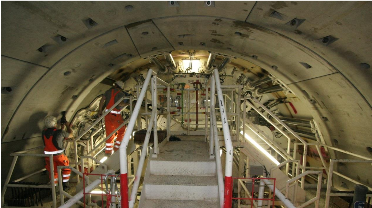
Figure 1-9: Assembly of a tunnel ring - different segments of the tunnel ring with the smaller keystone at the top
