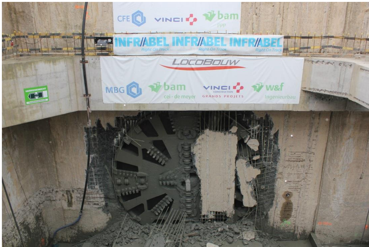
Figure 1-11: Tunnel Boring Machine 1 (“Wiske”) reaches its destination point at the arrival shaft
