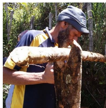
Figure 5.54. Placing the roof beam.
