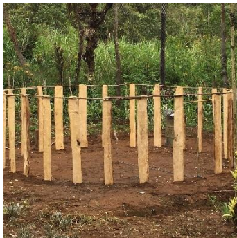
Figure 5.23. Ready for cladding.
