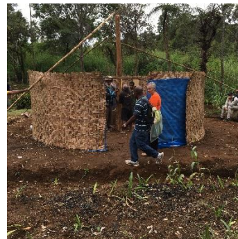
Figure 5.27. Aligning centre post.
