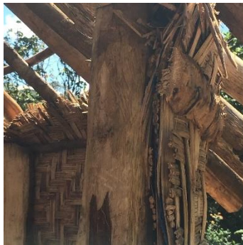
Figure 5.29. Rafter connection.
