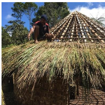
Figure 5.42. Thatching the roof.
