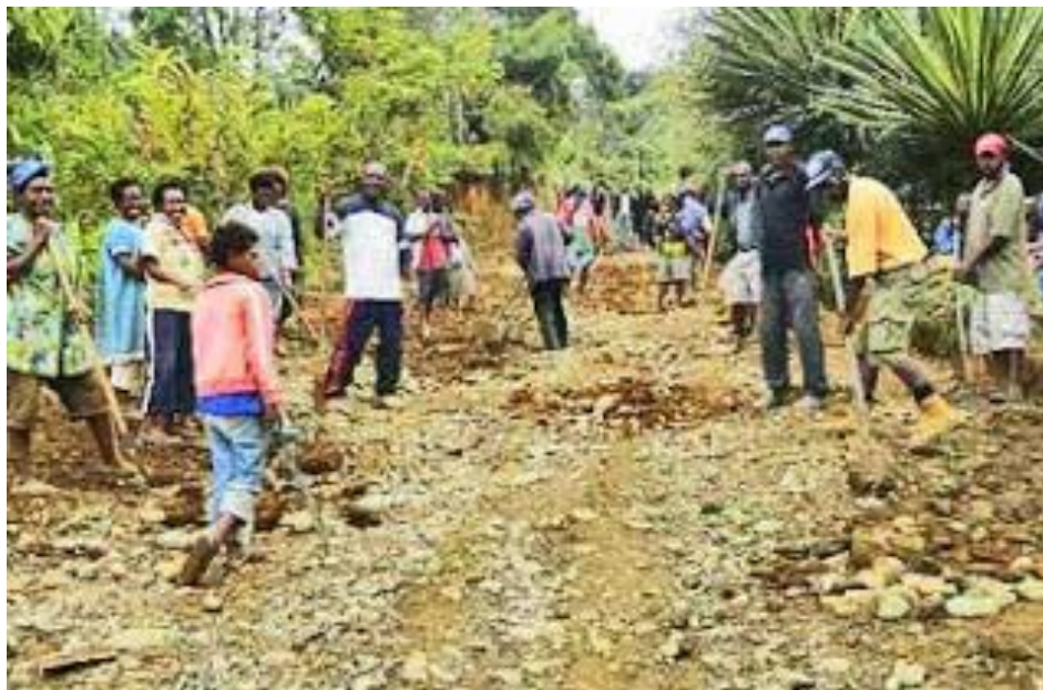
Figure 5.4. Mt Hagen to Mt Kuta road construction. Source: Poiya (2013).
