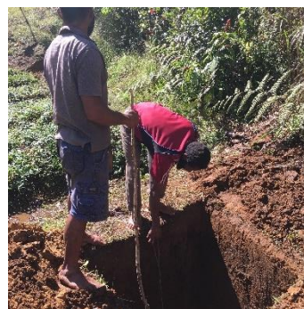
Figure 5.51. Digging the pit.
