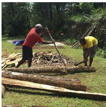
Figure 5.15. Splitting logs for posts.
