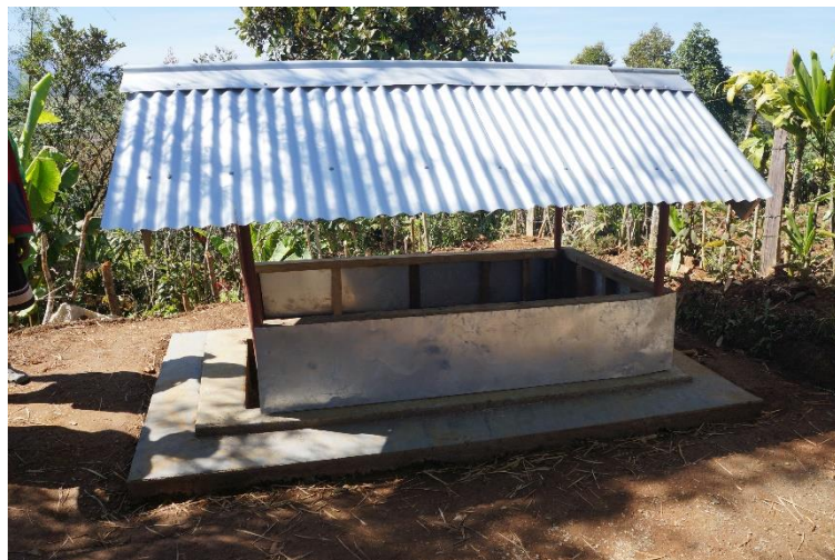
Figure 5.5. Newly constructed funerary house. Source: author (2016).
