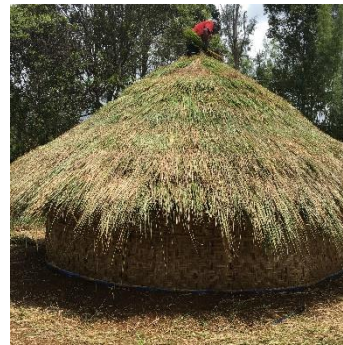
Figure 5.45. Ridge capping.
