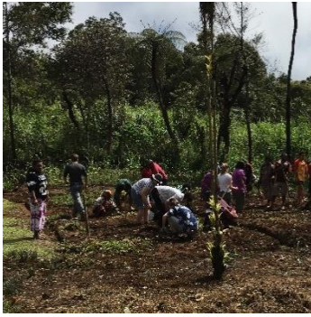
Figure 5.12. Clearing the site.
