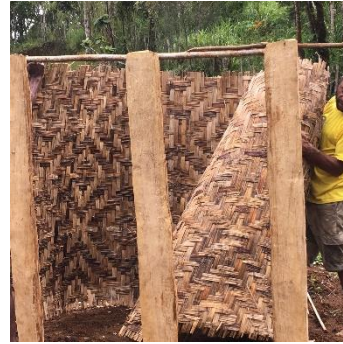
Figure 5.24. Internal lining.
