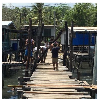
Figure 5.81. Ocean pile driving.
