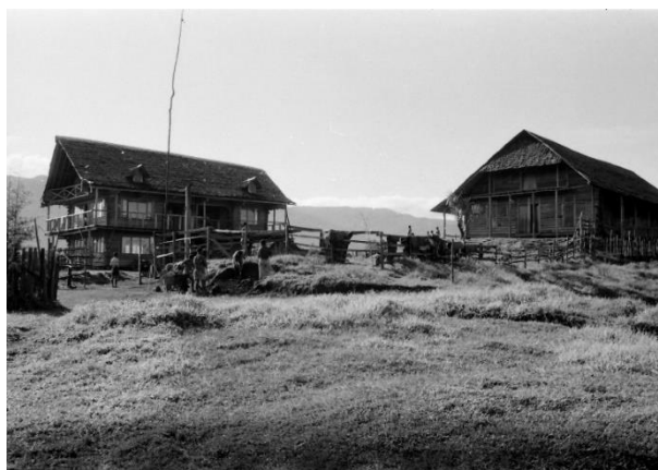
Michellod Log Cabin and Church, Kosipe, PNG ca.1970s. With permission: Hope (2009b). No nails were used in the construction of these buildings.
