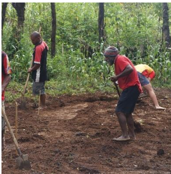
Figure 5.13. Levelling the site.
