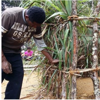
Figure 5.55. Wall cladding for WC.
