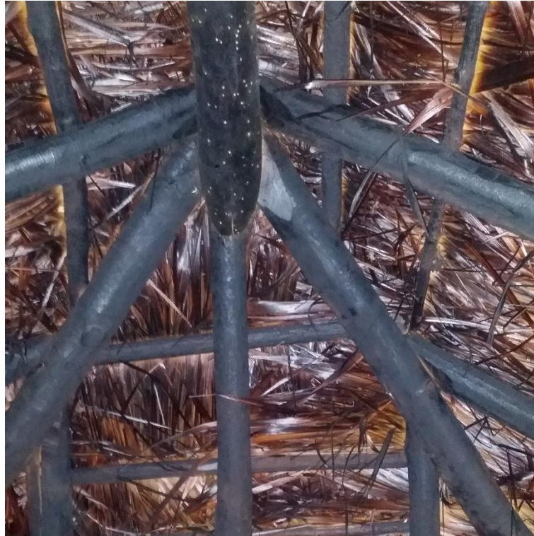
Figure 5.74. Roof framing inside Kuipa's house.
