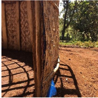
Figure 5.28. External cladding.
