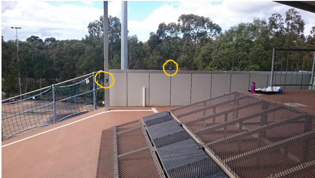
Figure 5-2 Camera placement on the SX ramp platform
