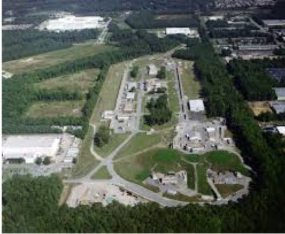
FIG. 5: Aerial view of the Thomas Jefferson National Accelerator Facility in Newport News, VA. The three experimental Halls can be seen in the lower right corner of the image.
