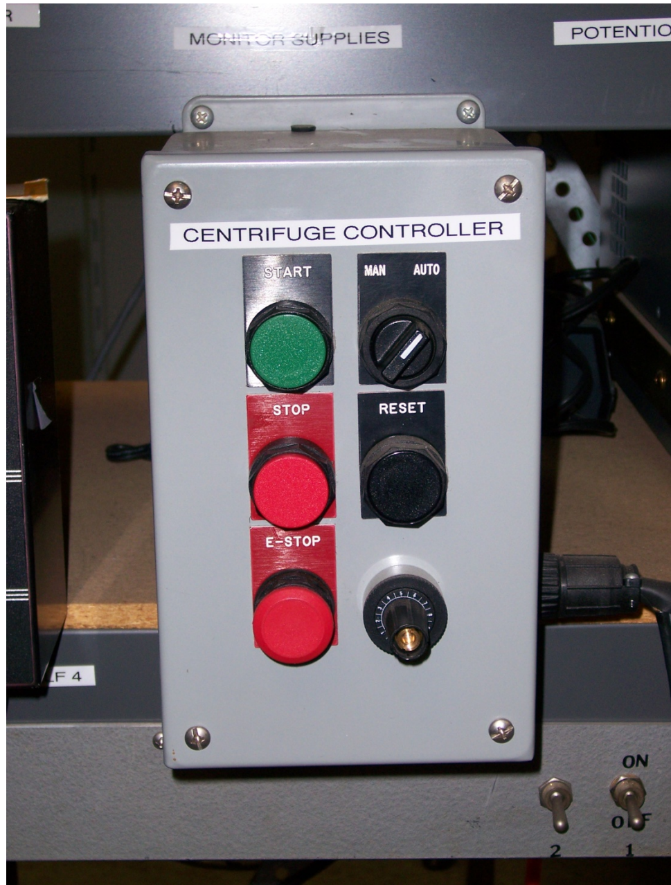
Figure A.2. Centrifuge table control panel box.
