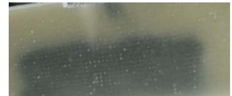
Composite patch side without crack
