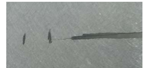
Aluminum structure side with crack
