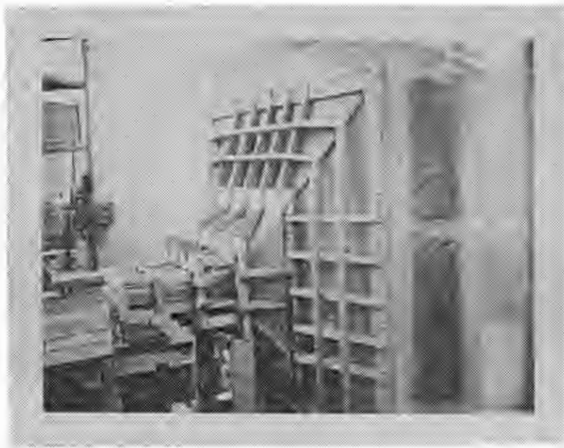
PLATE D-2. WIND TUNNEL: PLENUM CHAMBER AND CONTRACTION (SIDE VIEW)
