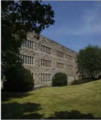
Figure 10. Norris Hall Classroom Windows, Grassy Side
