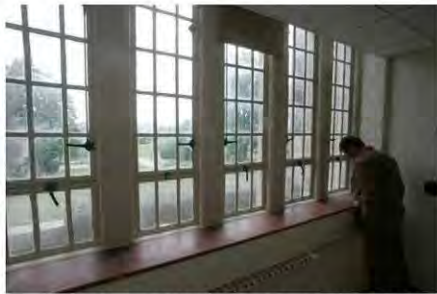
Figure 11. Typical Set of Windows in Norris Hall
