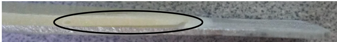
Figure 9. Delamination at the end of sample 4
