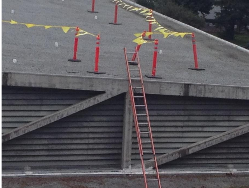
Figure 28. Safety setup at the work area entry point atop King Hall.
