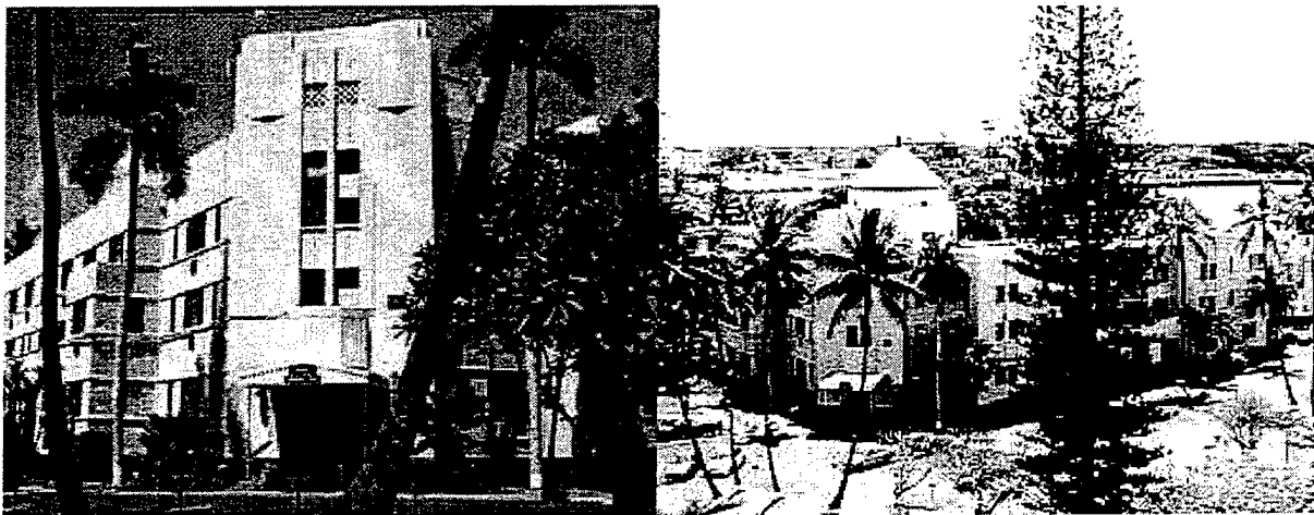
Figure 3. Lockwood Hall is one example of Bachelor Officer Quarters (BOQ). It is located on the submarine base in Pearl Harbor, Hawaii. Lockwood Hall, the Naval Station BOQ (BOQ 1315), and Makalapa BOQ (BOQ 372) on the Commander-in-Chief Pacific Fleet (CINCPACFLT) compound are all located within a five mile radius. Regionalization reduced infrastructure by combining the responsibility for all BOQ’s under one command. [U. S. Navy photos]
