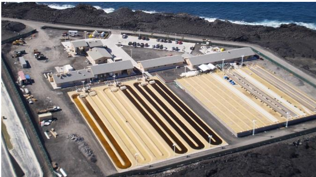
Figure 36. Algae farm demonstration facility in Kona, Hawaii utilizing hybrid growth method with photobioreactors (right) and open pond systems (left) (From Cellana 2013).
