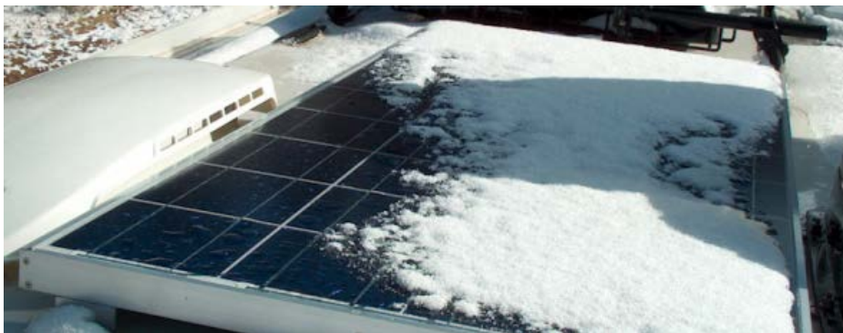
Figure 1. An example of a severely obstructed panel. Note the four panels completely unobstructed (From [18]).
