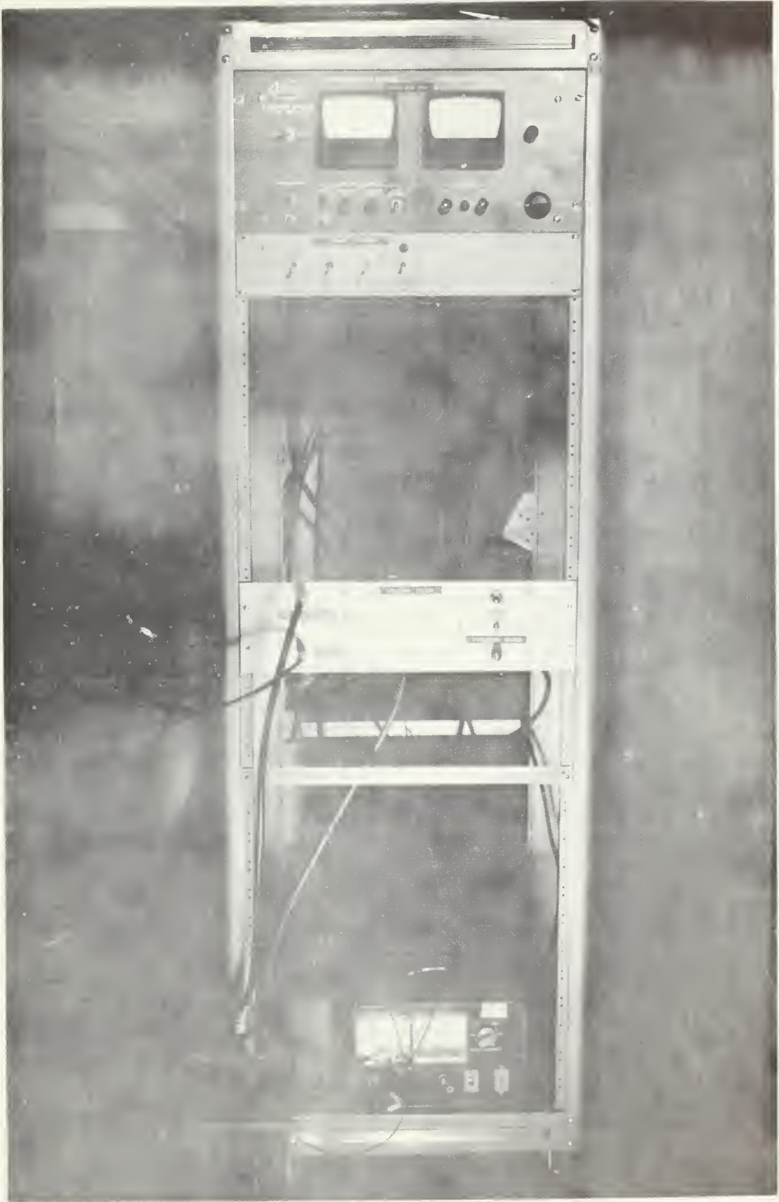
VACUUM CONTROL PANEL PULSED POWER SUPPLY AND TRANSFORMER FIGURE 4
