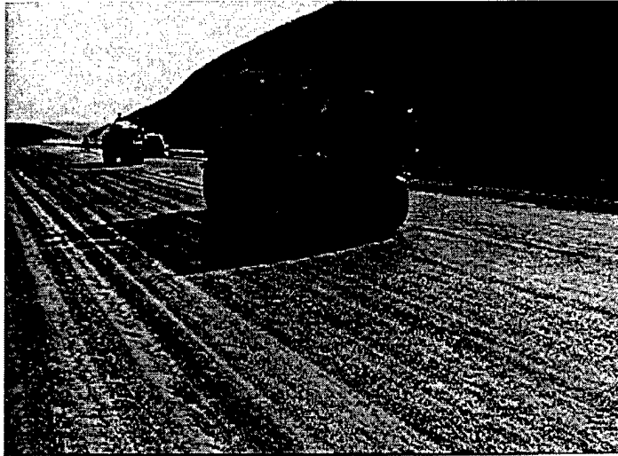
Fig 2.4 Consolidation of a G1 base layer in South Africa (photo courtesy of Kobus van der Walt, South African National Roads Agency)
