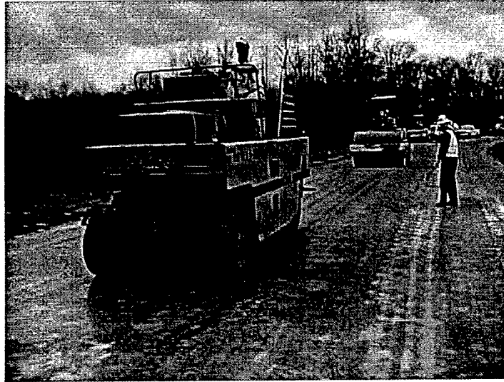
Fig. 2.7 Slushing of the GAB base in South African test section in Georgia (photo courtesy of Dwane Lewis, Georgia Department of Transportation)
