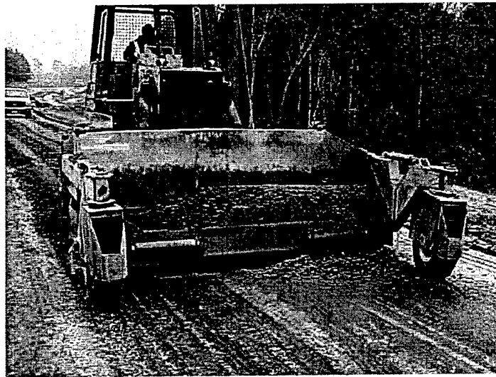
Fig. 2.6 Construction of the GAB base in Georgia (photo courtesy of Dwane Lewis, Georgia Department of Transportation)
