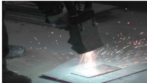
Figure 2.1 - Thermal spray application (From Thermion, Inc.)
