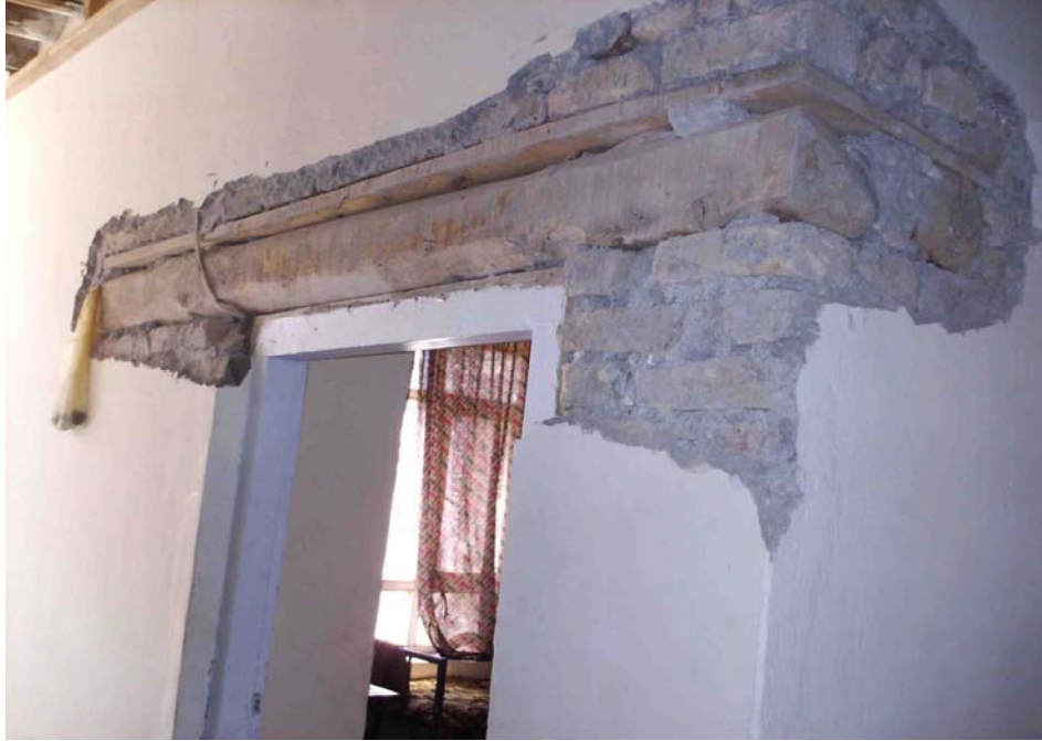
Photo 2. Interior Look at Roof Structure Showing Brick Wall Structure 296
