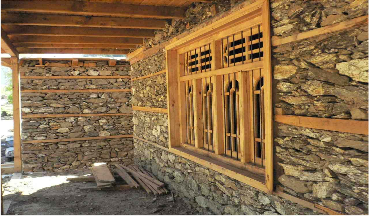
Photo 11. Close Up of Wall and Window Construction
