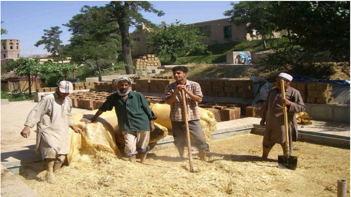
Photo 16. Mixing the Traditional Clay and Hay Wall and Roof Coverings
