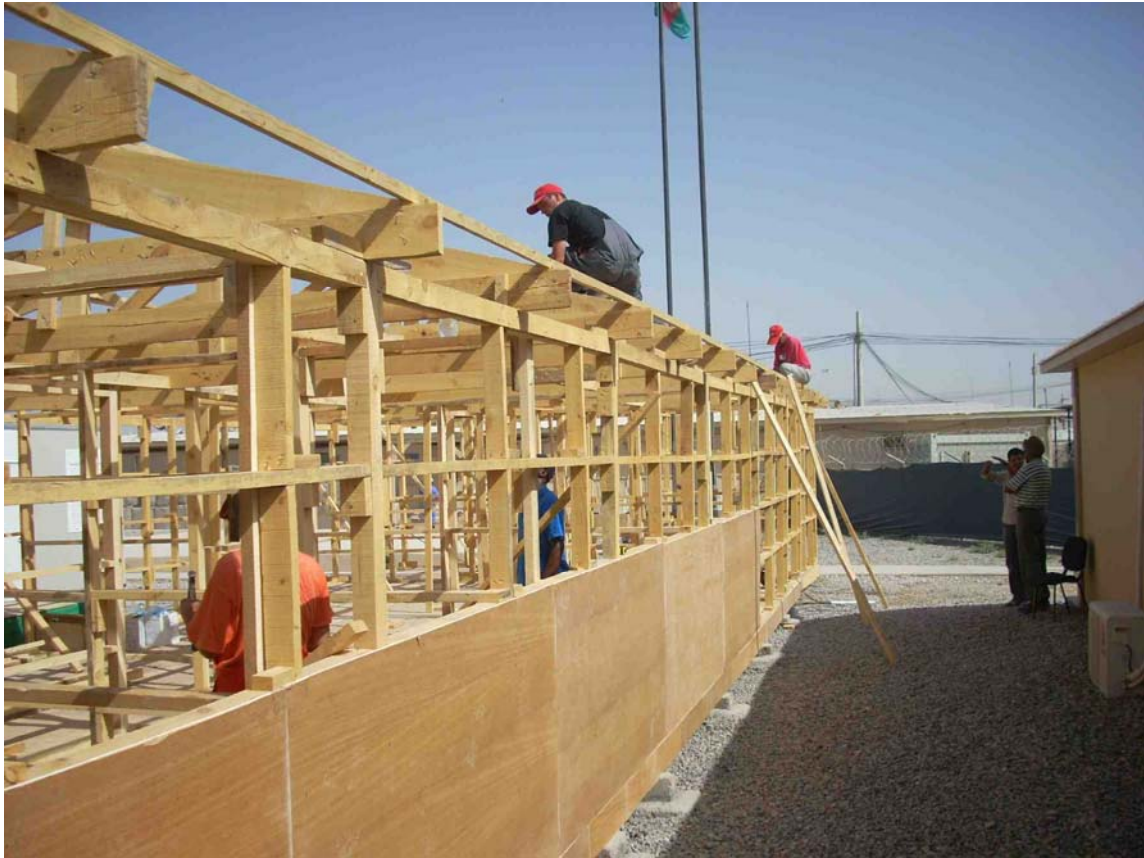
Photo 17. Typical Wooden Structure Built throughout the Country
