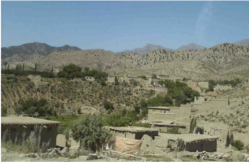
Photo 3. Flat Roof Construction in Khost 297
