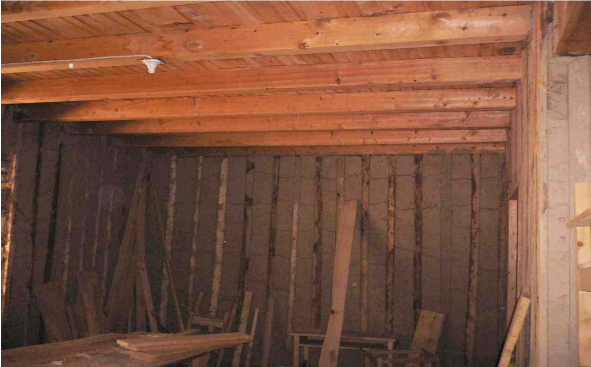
Photo 10. Interior Room Construction, Notice the Tongue and Groove Ceiling
