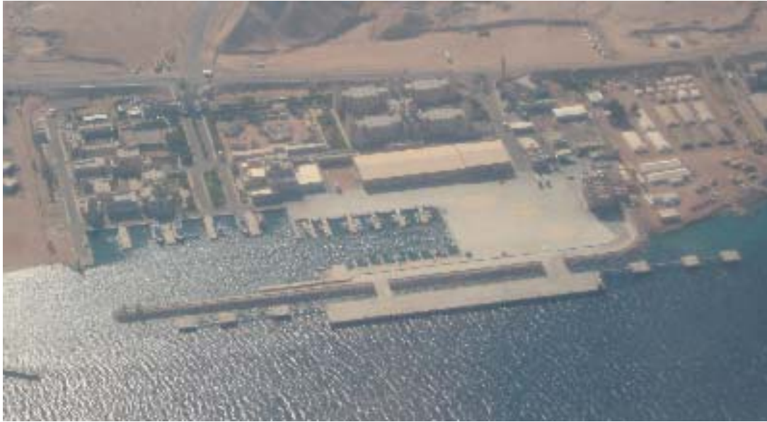
Figure 7. This is an aerial view of the Royal Jordanian Naval Base in Al'Aqaba. Joran, taken from a plane in July 2008.
