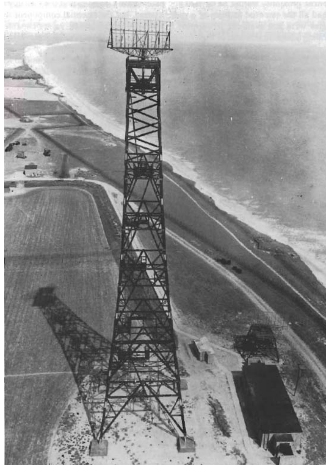
Figure 17. The Chain Home Low Station at Hopton on the Norfolk Coast (From Browne and Thurbon 1998, 14)
