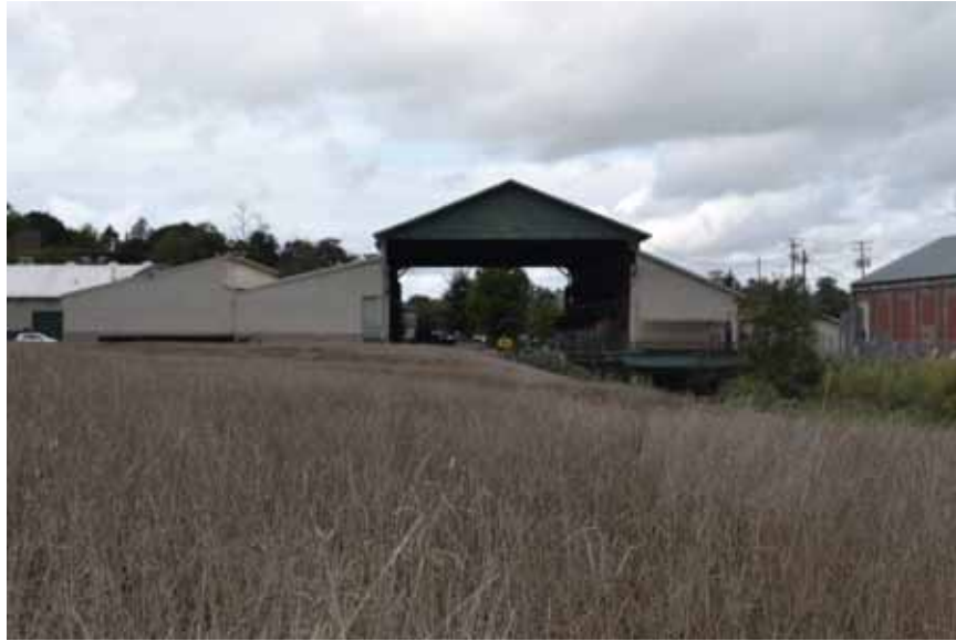
Figure 5: Existing crane shed.
