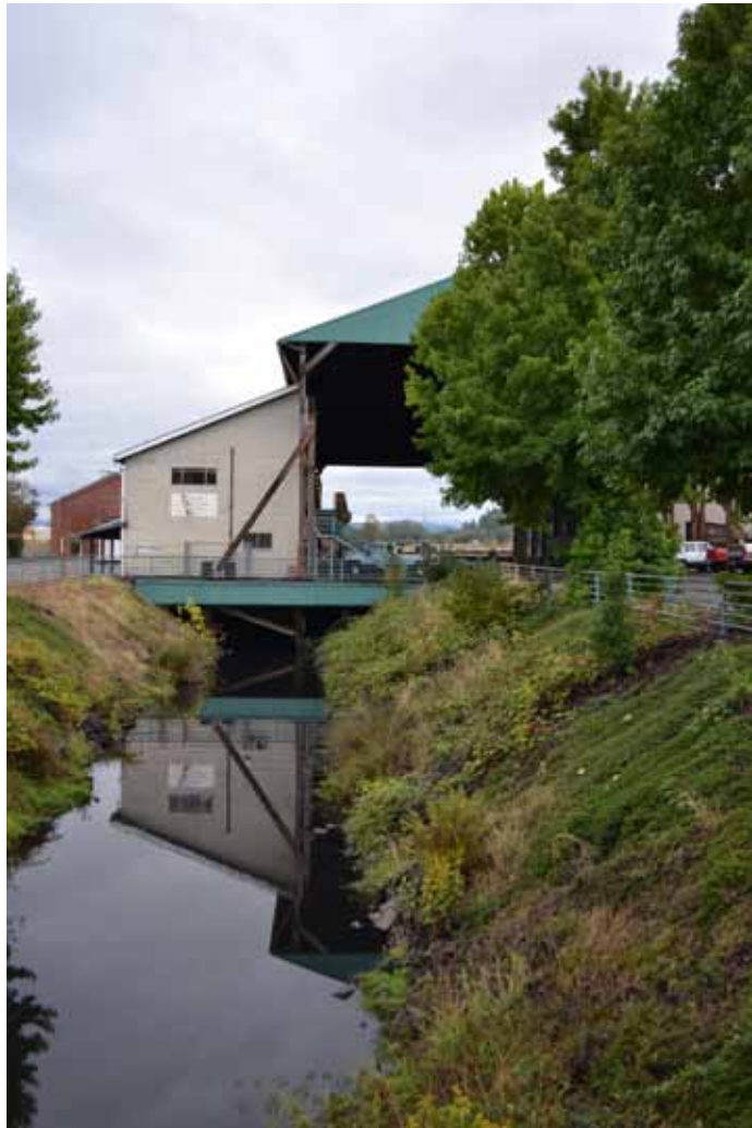
Figure 10: Millrace flowing under the crane shed
