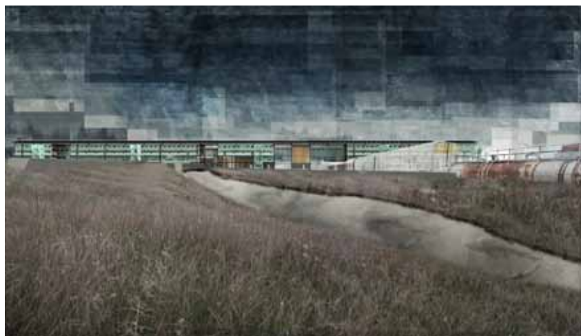
Figure 52: Cohen, South facade
