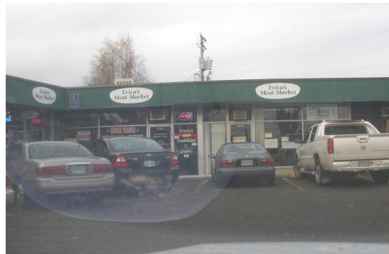
Figure 28: The small shops along Main Street and the buildings they occupy may not give the best representation of their offerings. Repainting the buildings and adding preventive measures would help beautify the building and neighborhood area behind it.
