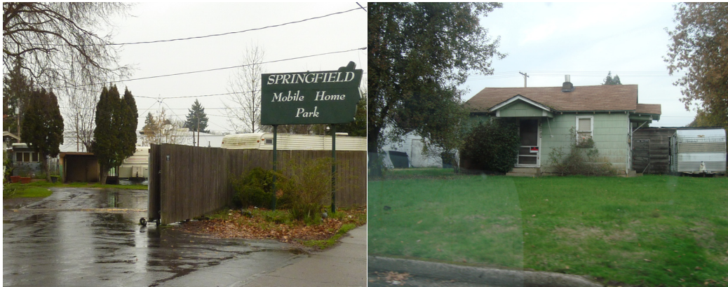
Figure 39: Springfield Mobile Home Park is a good example of centrally located low-income housing.
